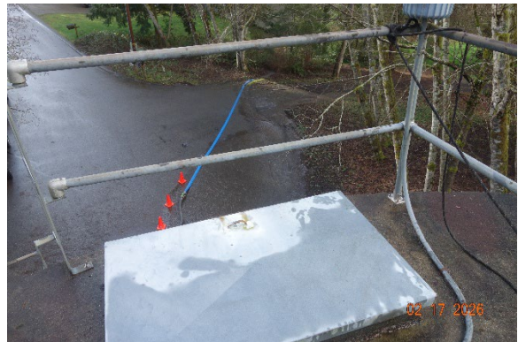
(#11) Access Hatch/Safety Railing
