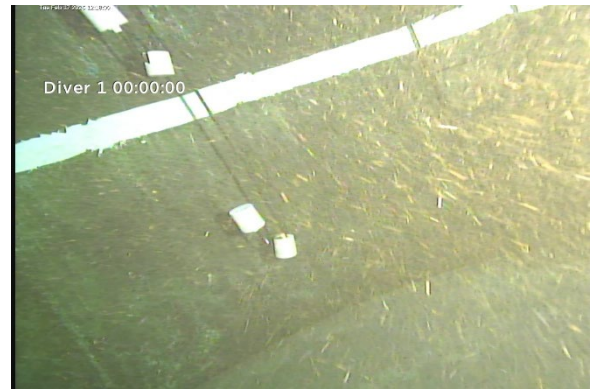
(#17) Wall Course Seam/Float
